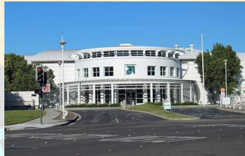
AMD Headquarters (Sunnyvale, California)
